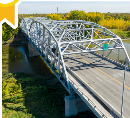
Kennedy Bridge Rehab - Grand Forks, ND
