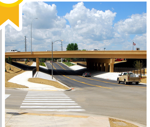
US 2 & 18th St W Underpass - Williston, ND
